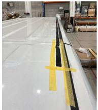
Primer Dry time (can be applied between  $5^{\circ}$  to  $40^{\circ}$  Above  $15^{\circ}$  10 min
